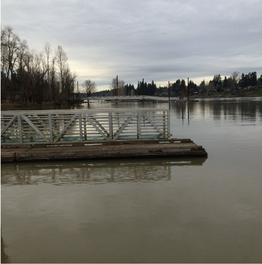
Photograph 9: Existing boat dock
