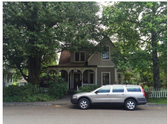
Existing house at 1831 5 th Ave.
