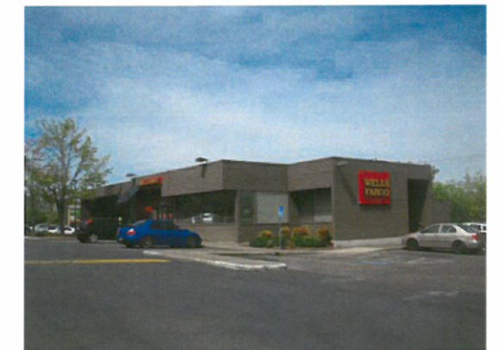
EXISTING IMAGE: Pad Building for Wells Fargo
