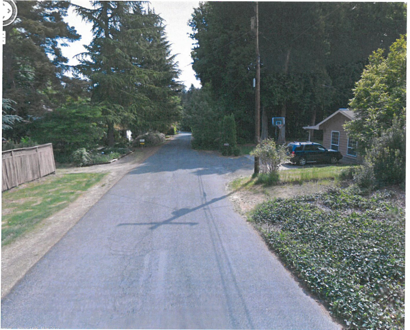
Looking east on Arbor Drive. You may be required to match this paved width for frontage of property being partitioned.
