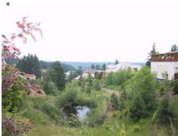
Figure 2.1. Storm Water Facility
