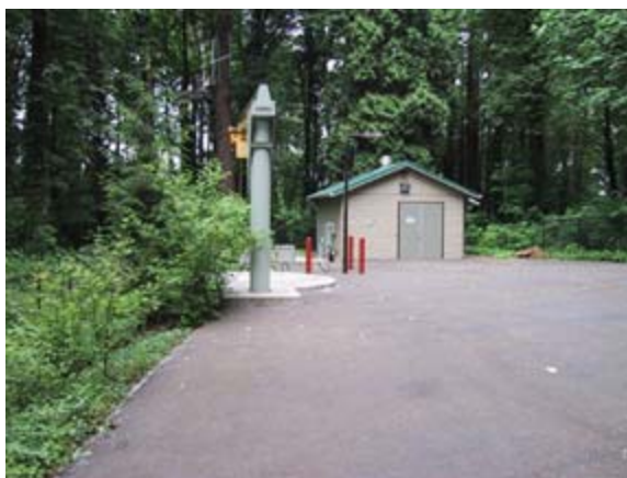
Figure 2.3. Sanitary Sewer Pump Station
