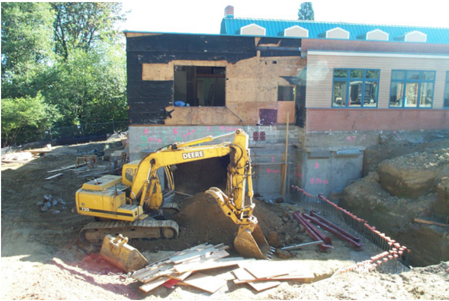
Construction during remodel
