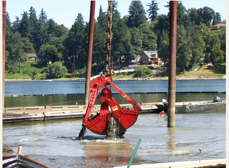
The dredging of the Cedaroak Boat Ramp keeps the waterway navigable and useable. Dredgings were placed in the river at a shallow depth to create warm water fisheries.
