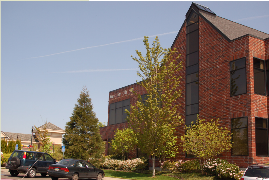
West Linn City Hall is located at 22500 Salamo Road.
