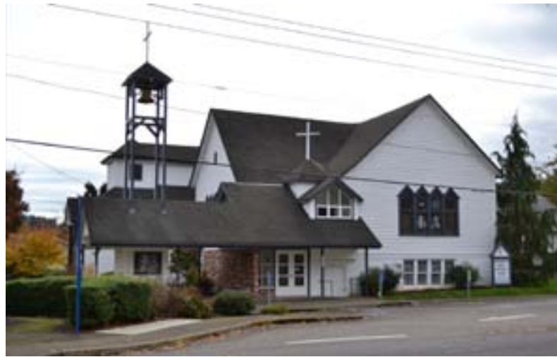
NOW: 2013 View of Willamette Methodist Church. Photo courtesy of Kendra Frankle, Rosemont Ridge Middle School.
