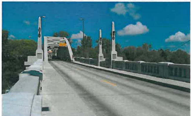
Recently rehabilitated Arch Bridge
