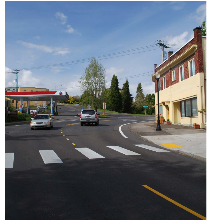
Willamette Drive with Broadway Street in the distance.
