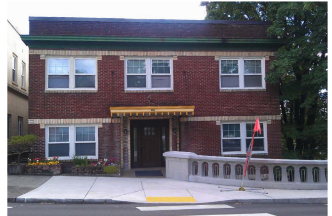
Historic building c. 1920
