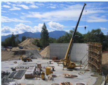
New 5.0 MG Reservoir AWWA D110 Type I Completed: 2014
