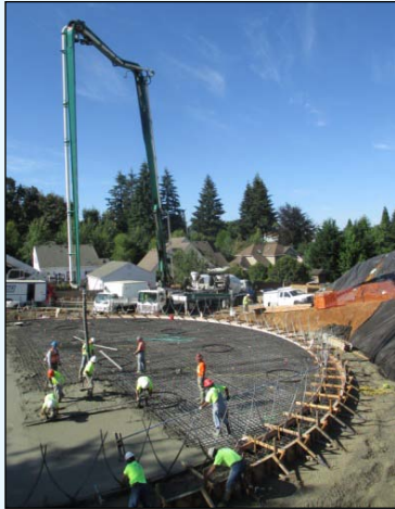
New 1.0 MG Reservoir AWWA D110 Type I Current project
