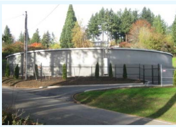
New 3.0 MG Reservoir AWWA D110 Type I Completed: 2009
