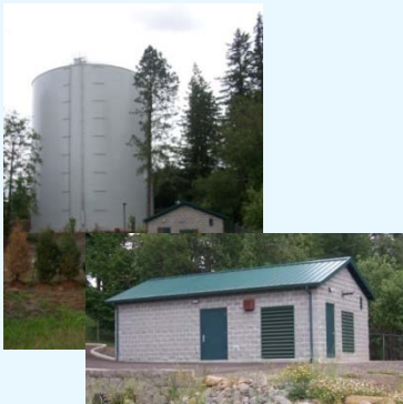
New Water Booster Pump Station
