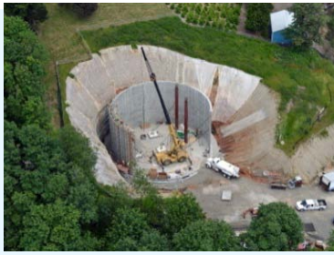
New 1.3 MG Reservoir AWWA D110 Type I Current project
