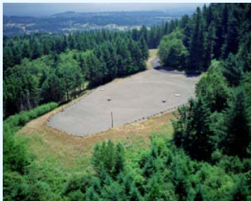
New 4.0 MG Reservoir AWWA D110 Type I Completed: 2005
