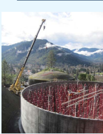
New 1.2 MG Reservoir AWWA D110 Type I Completed: 2011
