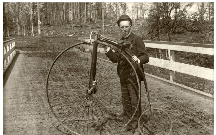
1895 photo of a high-wheeler bicycle on the West Linn end of the Oregon City suspension bridge. Photo courtesy of Old Oregon Photos.
