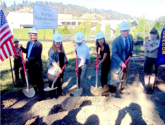
City Council at the ground breaking for the new Police Station
