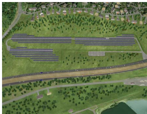
Aerial view of the potential West Linn site for the "Largest Solar Highway Project in the World"
